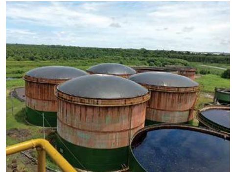
Anaerobic Digester Tanks (Maujaya CPO Mill)
