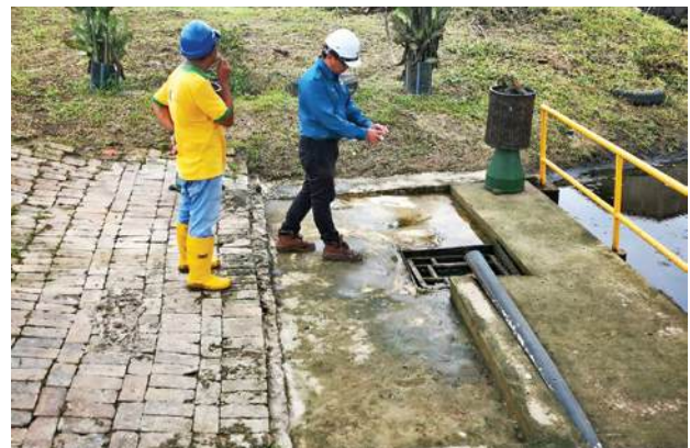
DOE inspection and record for the discharge point
